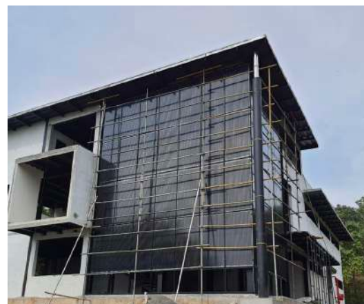
Fig. 4.11 Curtain wall under construction. Source: TopSun
