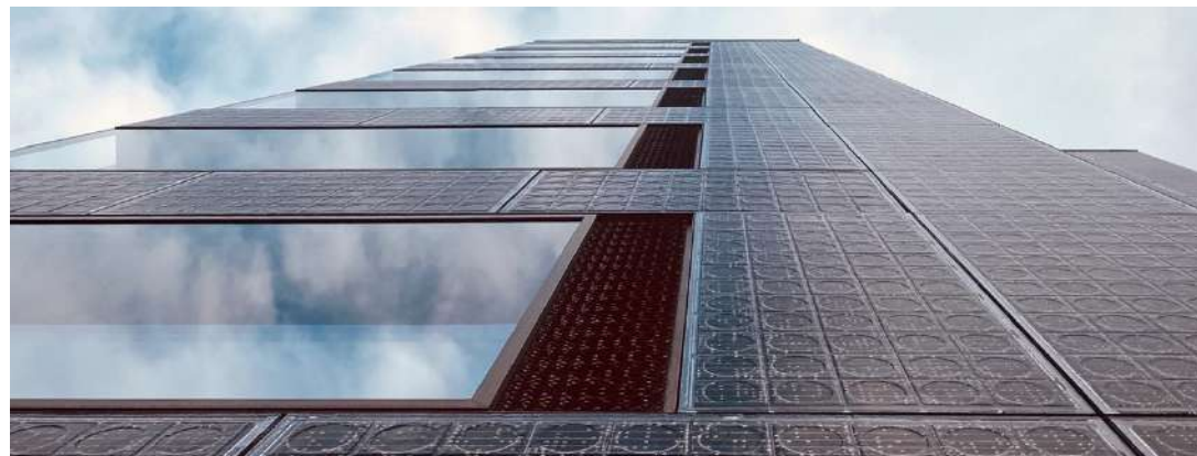
Fig. 3.2 Office for Environment and Energy (AUE), Basel. Source: solarchitecture.ch.
