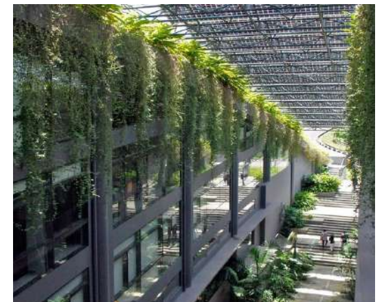
Fig. 4.15 Canopy, interior view. Source: Stapati.
