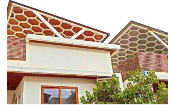
Fig. 4.8 View of the PowerRoof. Source: SunEdison.
