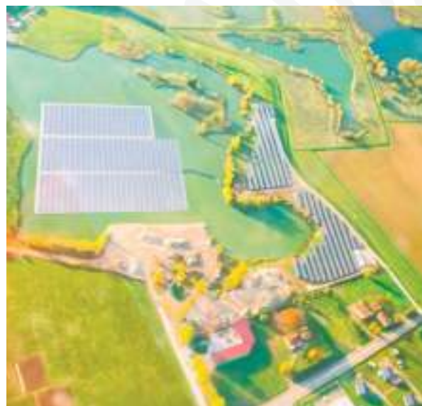
Amarenco's Floating PV site in Montpezat, France.
