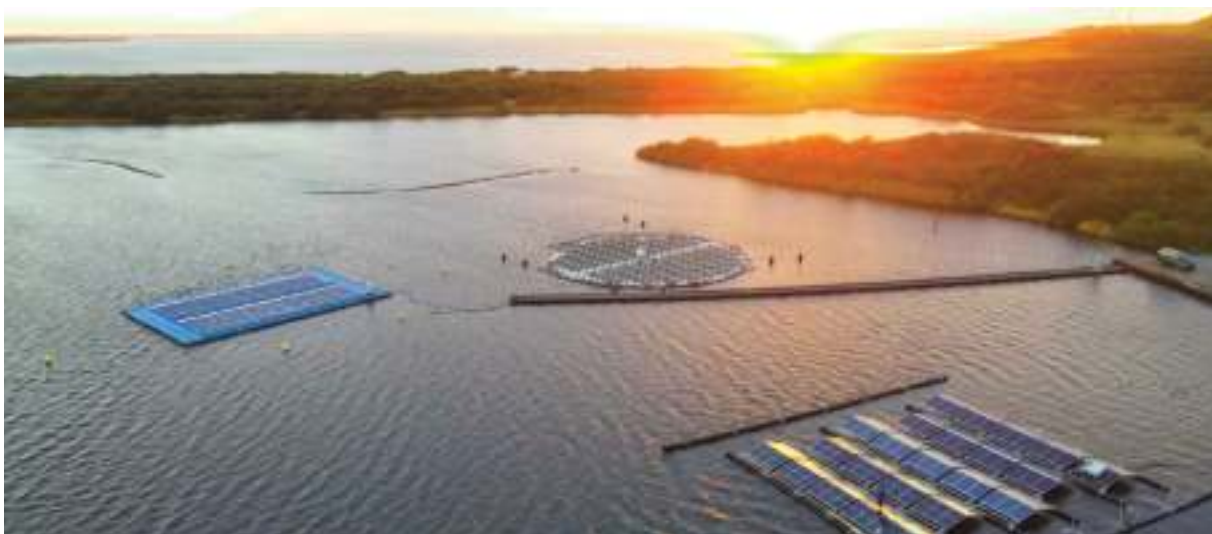
FieldLab 3 FPV systems located North-East side of Lake Oostvoorne.
