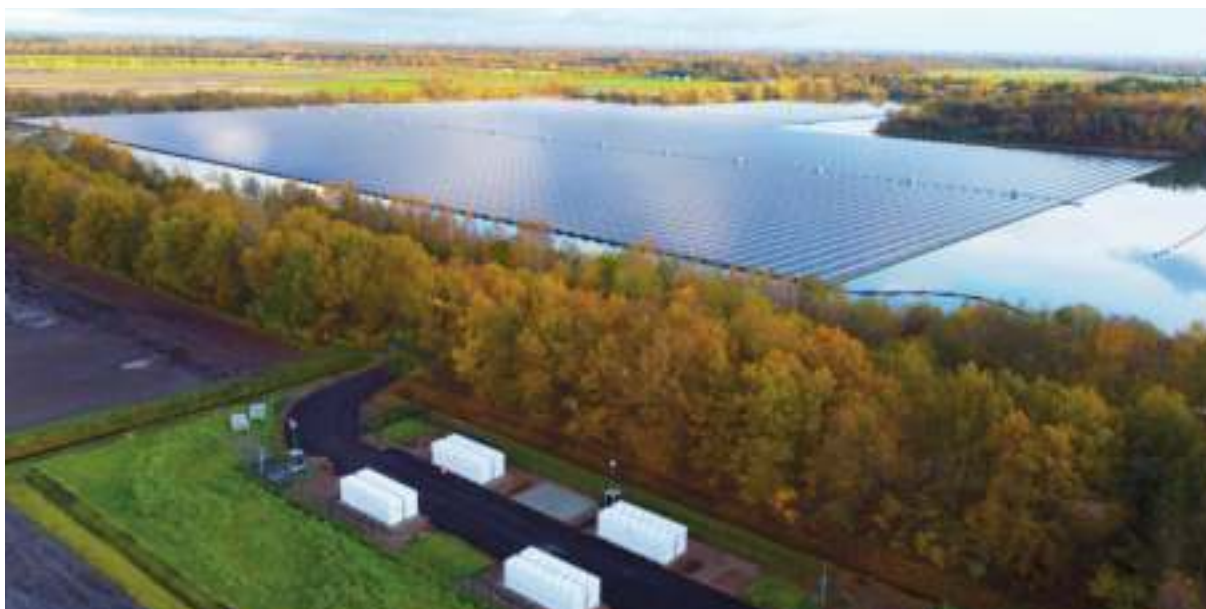
Floating PV site co-located with battery storage.
