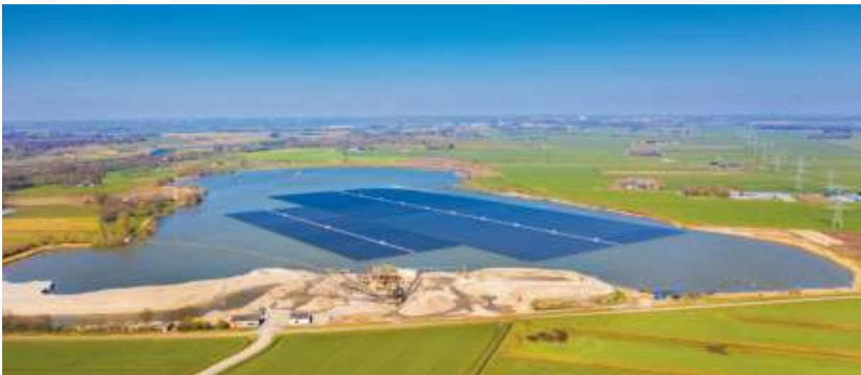
Bomhofsplass Floating solar park landscape.
