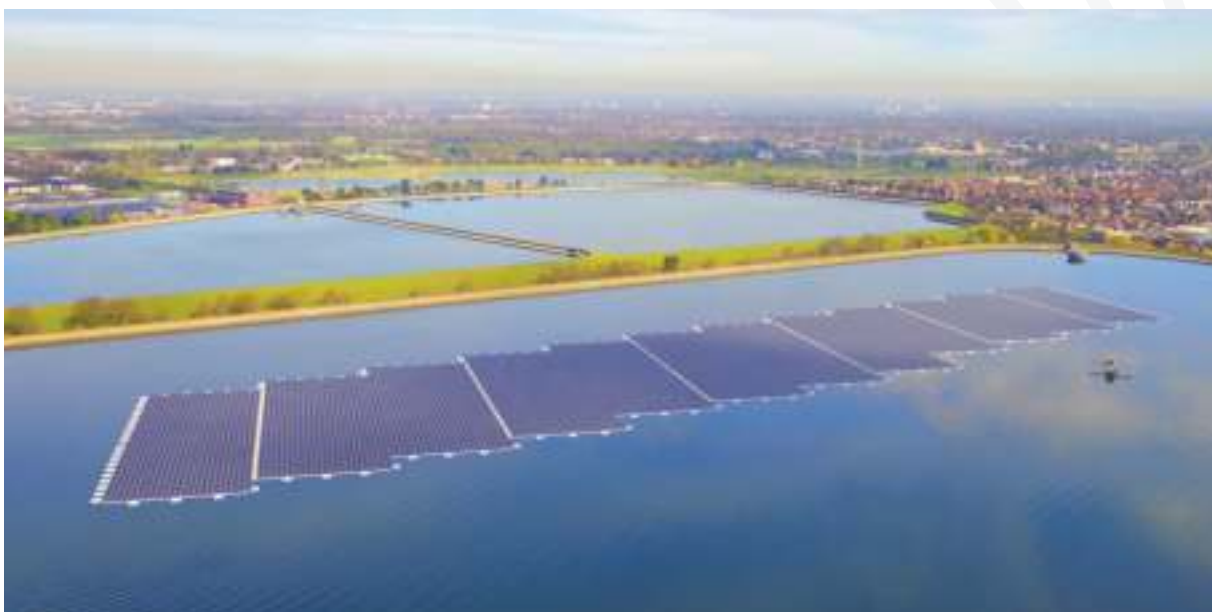
6.3 MW floating solar installation on the Queen Elizabeth II reservoir.
