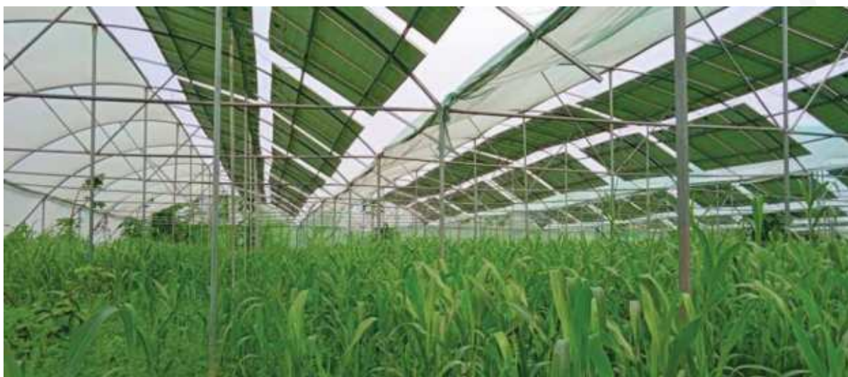
Plant B, Indra Solar Farm, Agrivoltaics plant, Tikamgarh, Madhya Pradesh. © Khare Energy Private Ltd.
