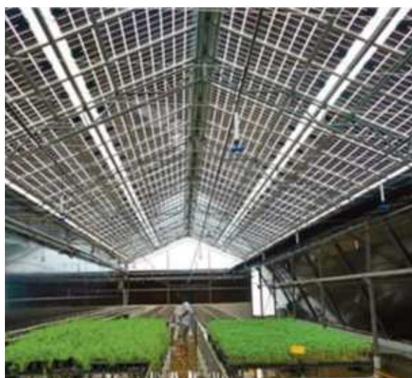
Greenhouse PV using Building Integrated Photovoltaic (BIPV) modules. © Jain Irrigation.
