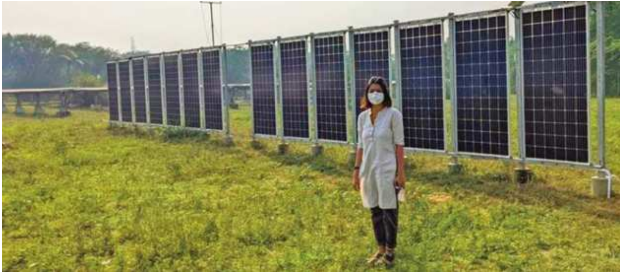
5 kWp pilot site with vertical bifacial modules. © National Institute for Solar Energy (NISE).
