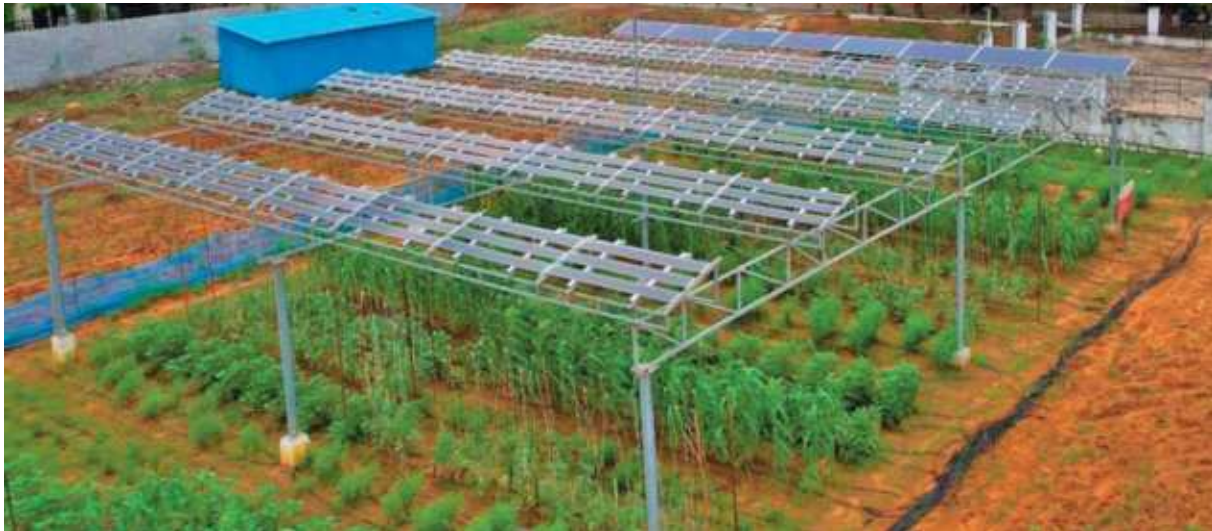
Semi-transparent PV panels installed at Seed Research and Technology Centre (SRTC), PJTSAU, Rajendranagar, Hyderabad. © Renkuba.
